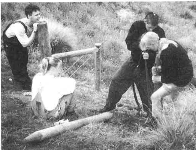
Holes for fence posts were dug by hand (David Blair)
